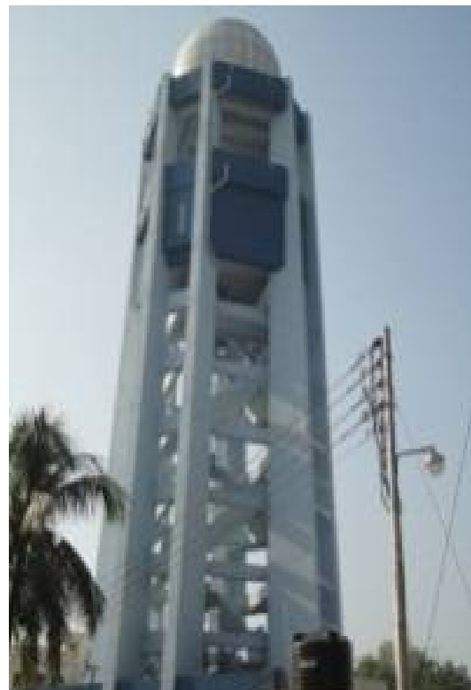
Meteorological Radar at Moulvibazar
